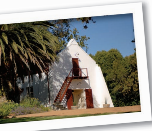
SACEMA is housed in the old wine cellar at Mostertsdrift.
